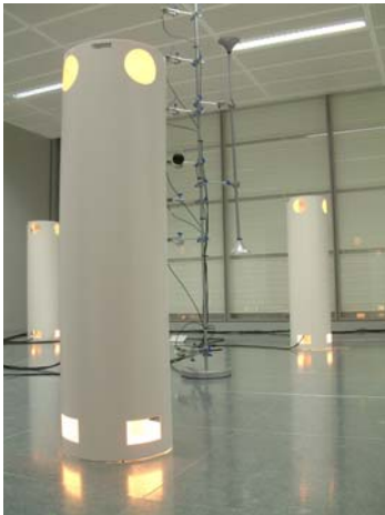
DIN man' representing occupant heat load in Frenger testing facility.
